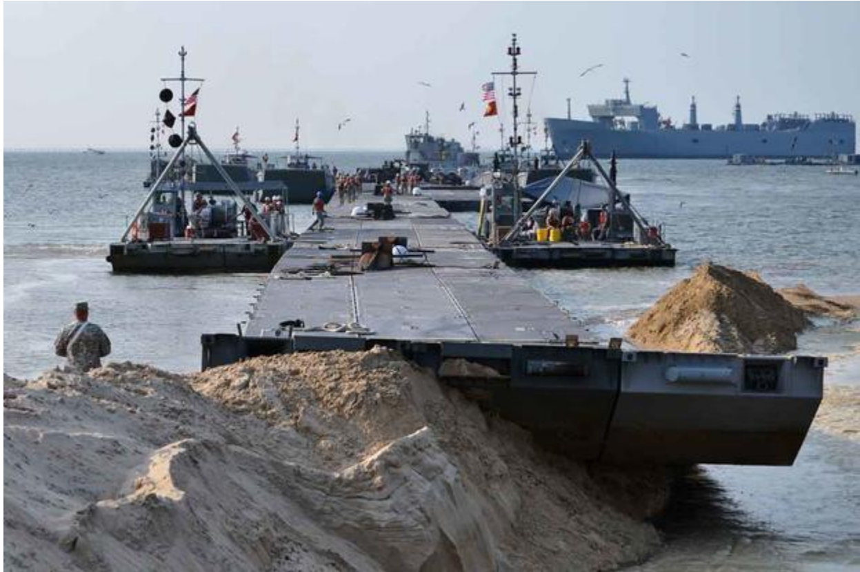
The Trident pier rests on the shore of Fort Story after an attempt to 'stab the beach' during the preliminary stages of the Joint Logistics-Over-the-Shore exercise, Aug.17, 2012. (Source: US Army, Defense Visual Information Distribution Service, Photo by Sgt. Edwin Rodriguez)
